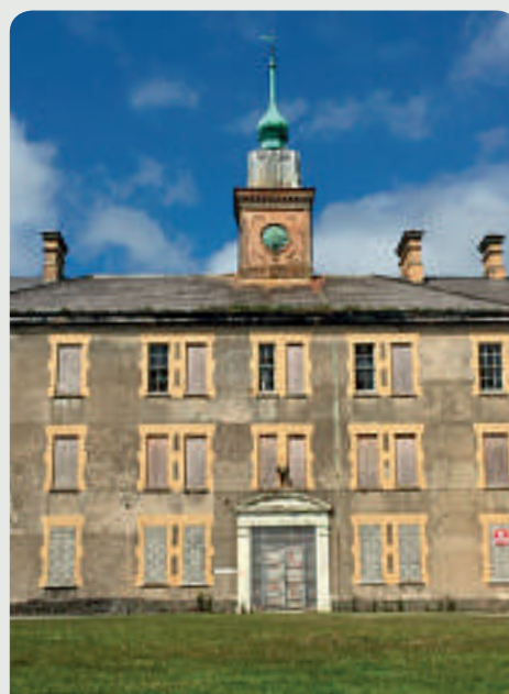
St Conal's Hospital, Letterkenny, 2015. Survey photo
